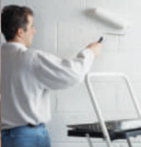
*Apply the second coat with a brush or masonry roller.*
