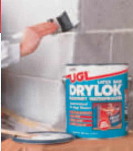
*Apply the first coat with a stiff bristle brush working thoroughly into the pores of the masonry surface.*
