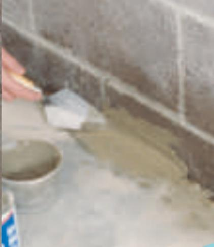
**Patch all holes and cracks with DRYLOK Fast Plug.**
