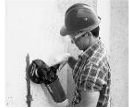
1. Clean surface along the crack. Blow out crack with dry and oil-free compressed air.
